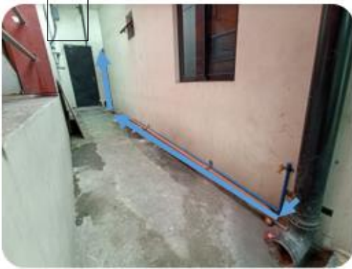
2. Back wash bleeding is diverted to the collection drain pipe to the collection tank located outside the water station and then accessed for use through the supply faucet shown in figure 4
