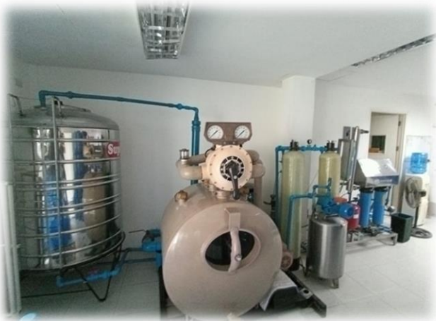
2. Back wash bleeding is diverted to the collection drain pipe to the collection tank located outside the water station and then accessed for use through the supply faucet shown in figure 4
