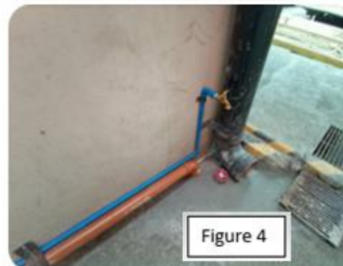
2. Back wash bleeding is diverted to the collection drain pipe to the collection tank located outside the water station and then accessed for use through the supply faucet shown in figure 4
