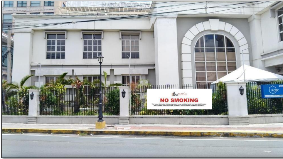
NO SMOKING BANNER AT SOUTH PERIMETER FENCE
