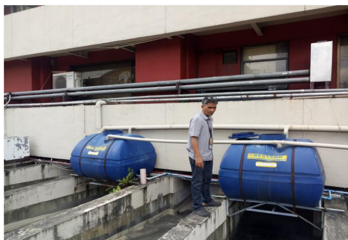
Mapúa Makati's rainwater collector tanks
