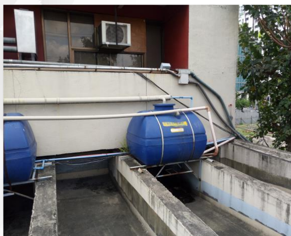
Mapúa Makati's rainwater collector tanks
